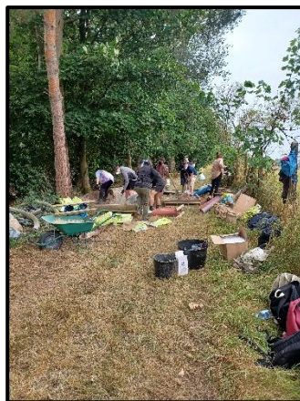
RS Group on a Wild Work Day filling sacks with sand and cement to reinforce the new track.
