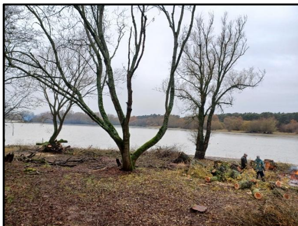
Clearing the area for the new accessible hide.
