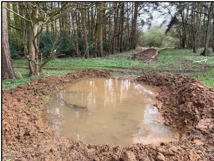
The drainage system on the west side of Scaldwell Bridge. A series of ponds, ditches and underground French drains were installed, while simultaneously creating temporary wet habitats that do not interfere with the path. © Andrew Cholerton.
